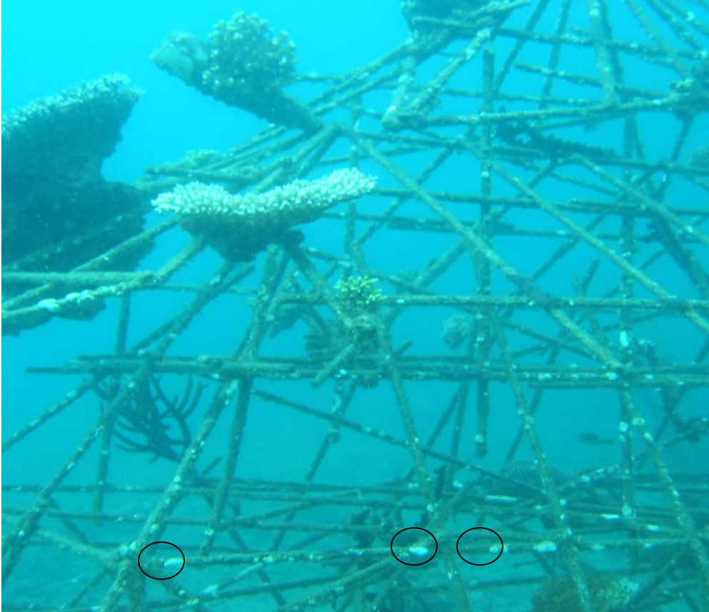
Figure 2: Pagoda biorock with calcium deposition (white spots) on the metal construction.
